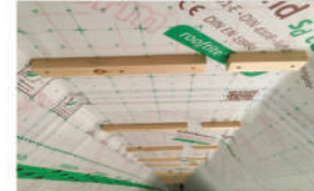
Fig 5.3 Gerband 586 sealing membrane overlaps
