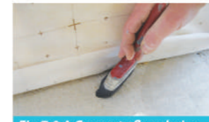
Fig 7.0 A Concrete floor being prepared by brushing dust/debris with paint brush.
