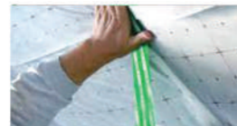
Fig 2.0 Sealing overlaps and repairing spots with Gerband 586.
