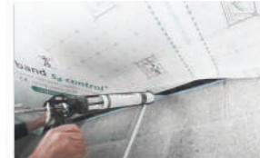
Fig 5.1 Sealing the membrane to masonry
