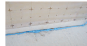
Fig 7.1 Fortax 6400 being applied, extra is used where surface is uneven.
