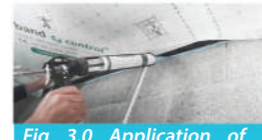
Fig 3.0 Application of Fortax 6400 Sealant to masonry wall.
