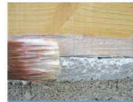
Fig 8.0 Primer being applied between wall and wall plate with paint brush.
