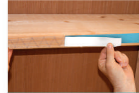
Fig 5.2 Fixing membrane to timber
