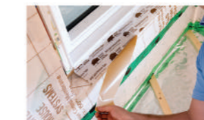
Fig 8.1 Remaining liner being released.
