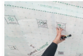
Fig 5.0 100mm overlaps before sealing overlaps
