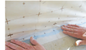
Fig 7.2 Membrane is gently pressed against sealant.
