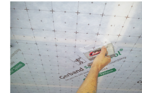
Fig 5.2 Stapling the membrane to timber
