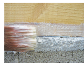
Fig 8.0 Primer being applied between wall and wall plate with paint brush.
