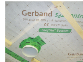
Fig 6.1 Sealing around services
