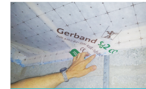
Fig 5.1 Sealing the membrane to masonry
