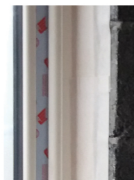
Fig 6.0 sealing window to masonry reveal
