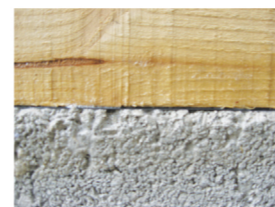
Fig 8.1 Primer is allowed dry before applying tape.
