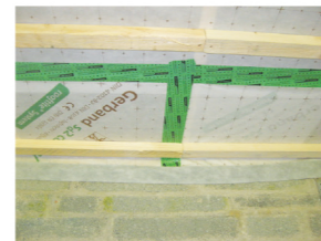
Fig 6.0 Sealing membrane overlaps
