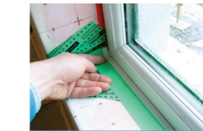
Fig 8.0 The installer has folded back the 12mm strip before removing the release liner
